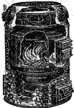
The Bovee furnace is the only furnace having a perfect forced Ventilating System, that insures pure air in every part of the house. The value of this forced ventilation cannot be over-estimated, especially in case of bad lungs or sickness.
